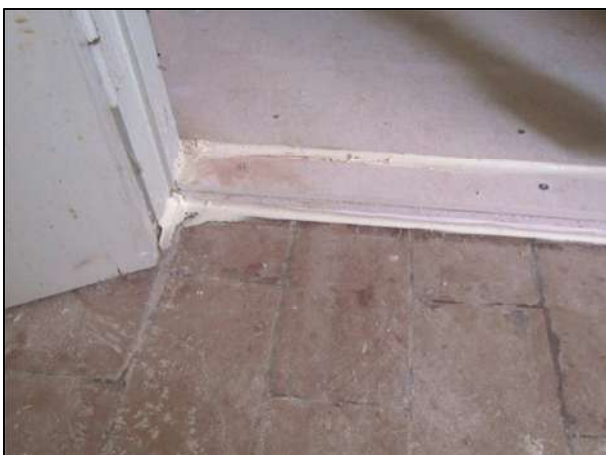
Photo of the covering at the access door
